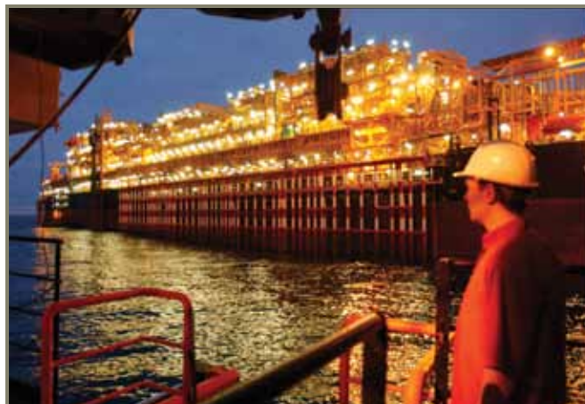
OFFSHORE SITE (APPLETON LIGHTING FIXTURES ON TOTAL GIRASSOL PLATFORM)
